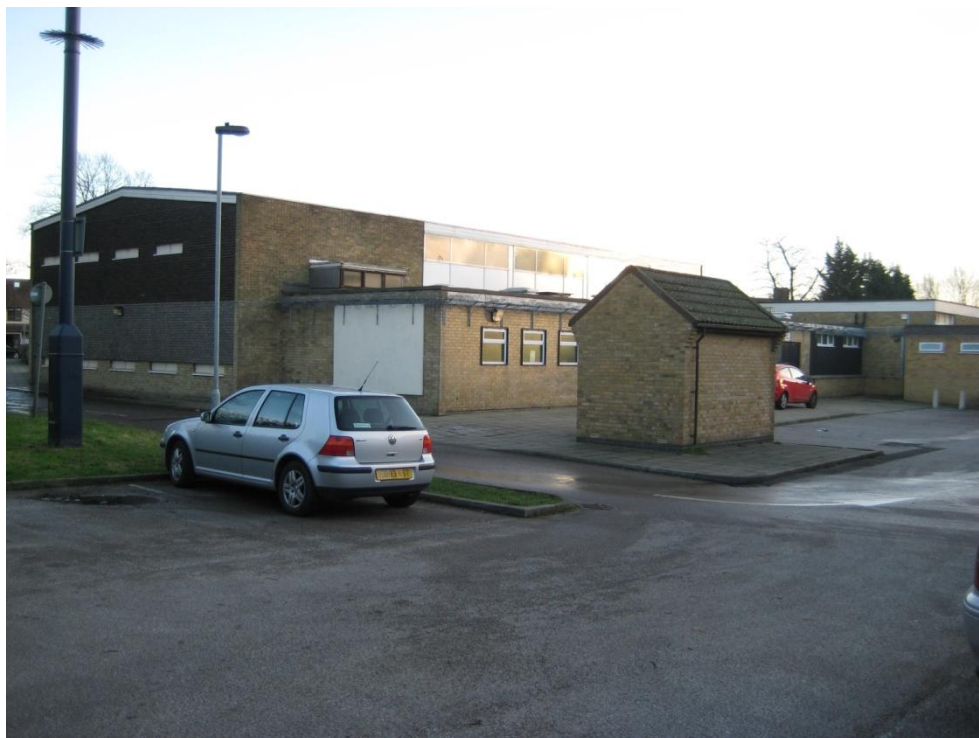
Community Centre (Rear)
